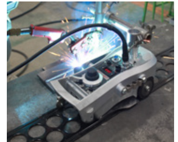
IK-12 NEXT straight welding
